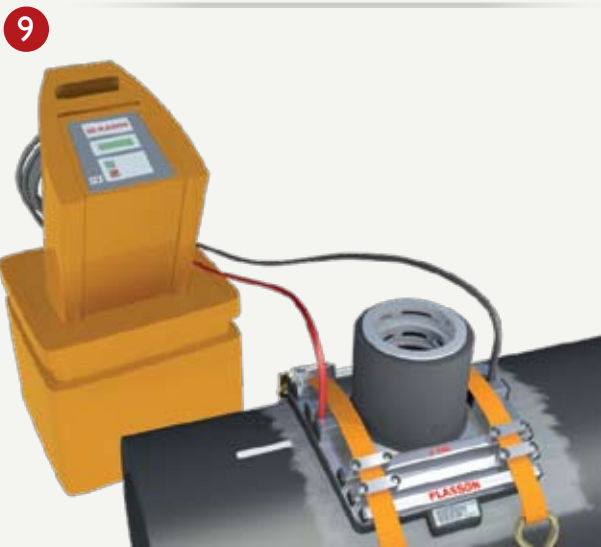
Fuse the fitting according to ElectroFusion procedures.
