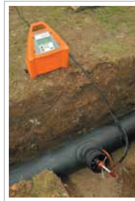
The Wastewater Saddle, with 160mm inlet Adjustable Coupler, offering an adjustable angled connection of up to 12°.
